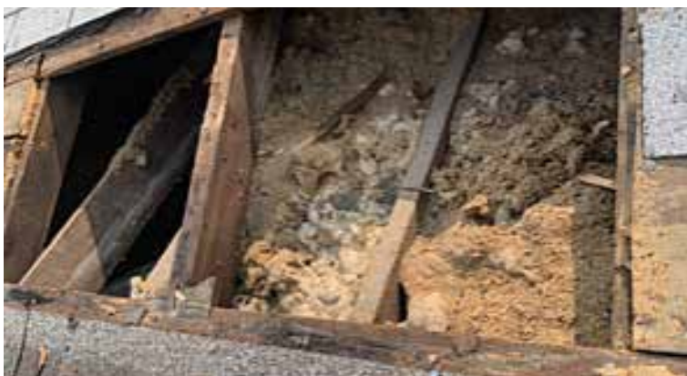
An Aug. 10 storm with hurricane-force winds caused much damage throughout Iowa.
